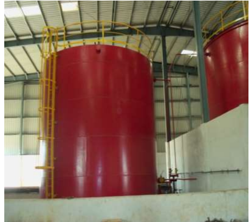
Liquid Storage Facility
