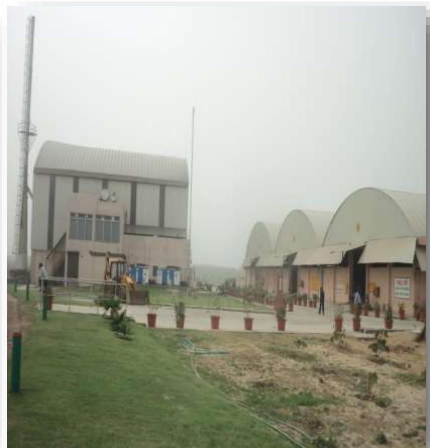
Overview of Facility
